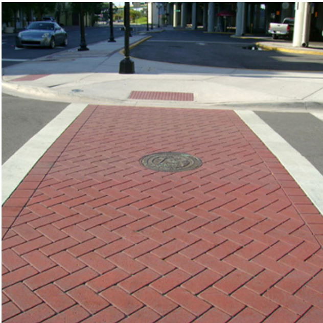
ENHANCED PAVEMENT - CROSSWALK PATTERNED STAMPED CONCRETE
